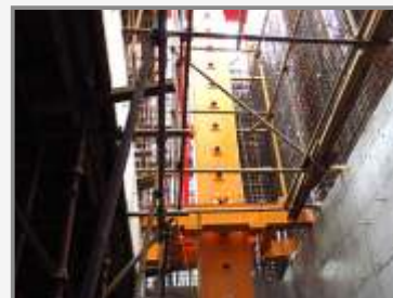
In lift shaft (Internal Climbing)
